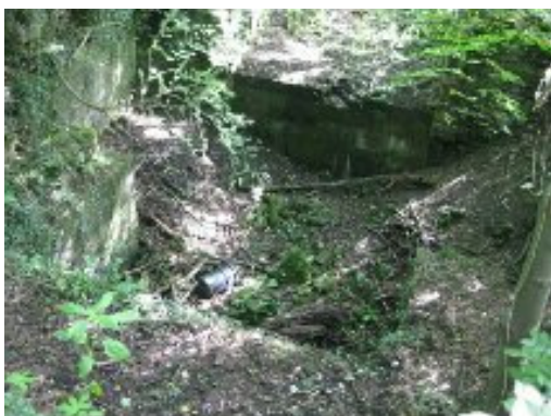
Wheel pit before clearing
